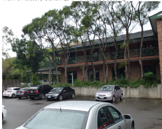
View of Administration Building
